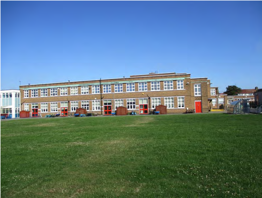
Rear elevation of main building
